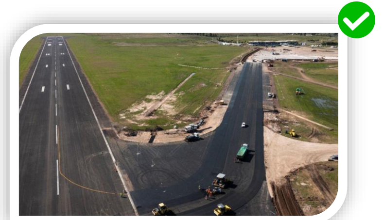
Resistencia Runway and taxiways repavement (May2023)
